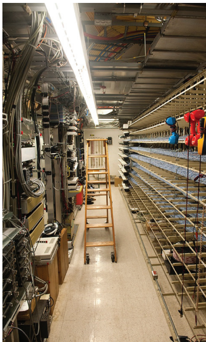
Wiring to connect to all campus phones
